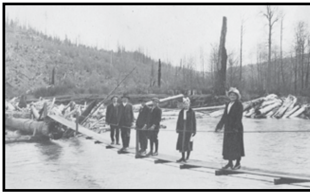
Temporary bridge across S. Fork at Nessel farm. Nessel barn and recently logged hill in background. ca. 1915.
