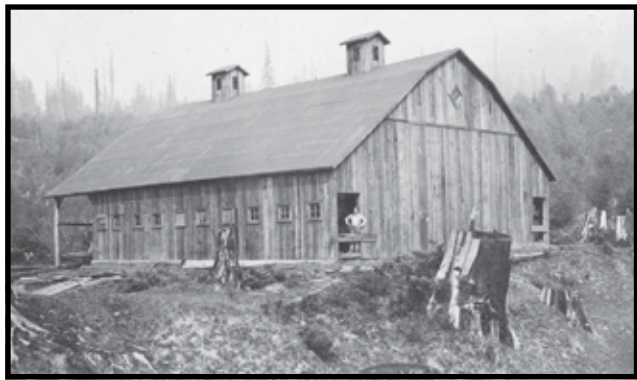
New barn nearing completion replacing original barn destroyed in flood. ca. 1920.
