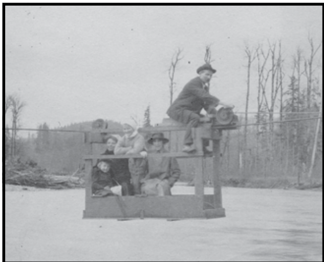
Lars operates hand-crank cable crossing over Nooksack River to trail for Nessel children to walk to Saxon School. ca. 1920.
